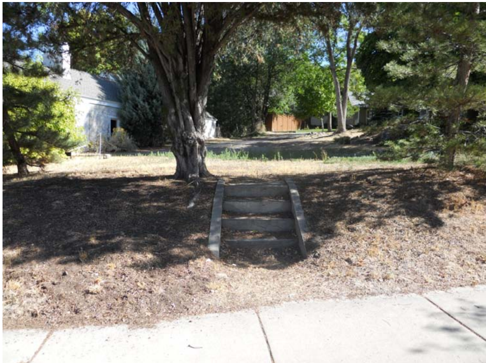
Remnant stairs at the front property showing evidence of a previous residence at the front of the lot.
